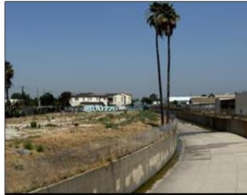
PHOTO 2: View looking west of the project site on the left and Eaton Wash on the right.
