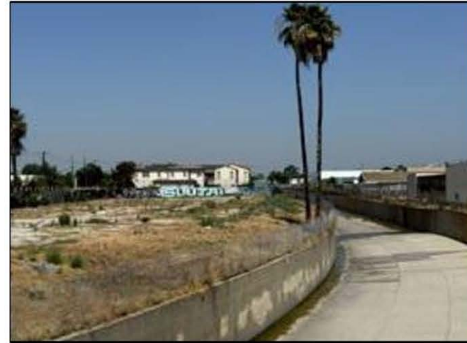
PHOTO 2: View looking west of the project site on the left and Eaton Wash on the right..
