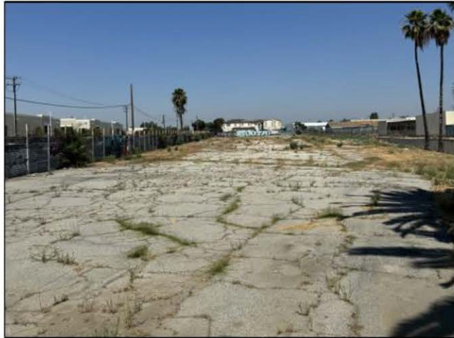
PHOTO 1: View looking west across the project site.
