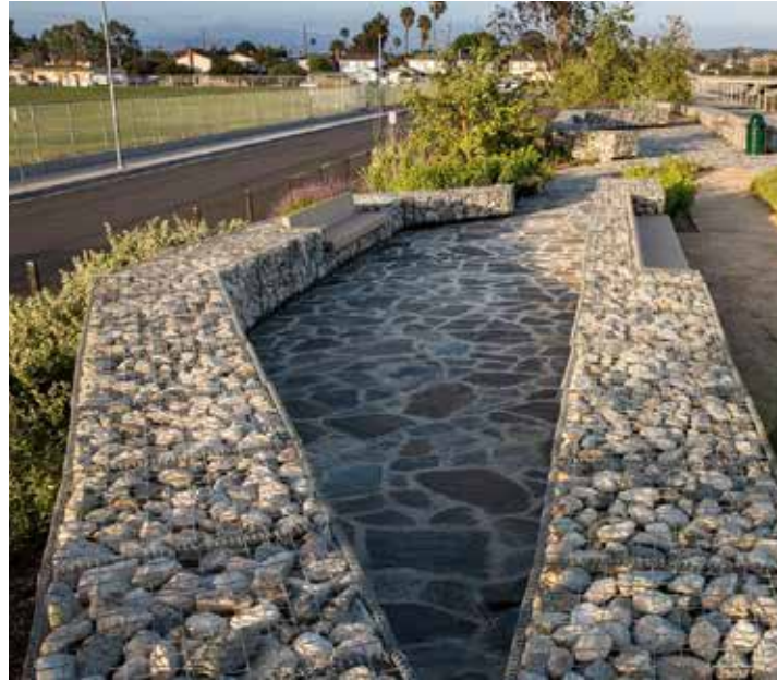
Gabion Seat Walls
