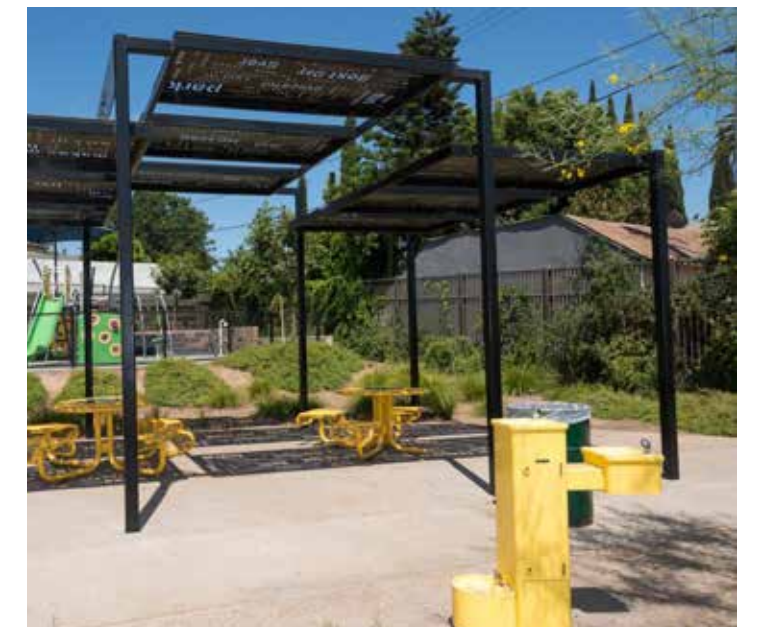
Custom Steel Shade Structure
