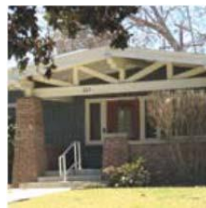
Exposed Beams/Rafters
