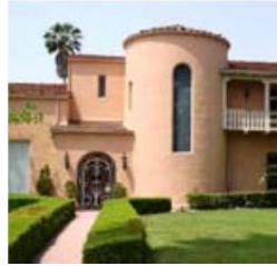
Complex Roof Forms
