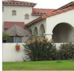
Arches and Arcades
