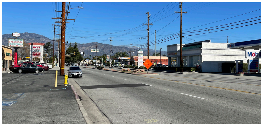
Existing roadway conditions along Peck Road and Lower Azusa Road
