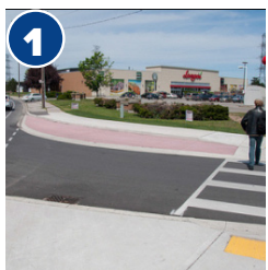
1 Corner Radius Reduction with Truck Apron
