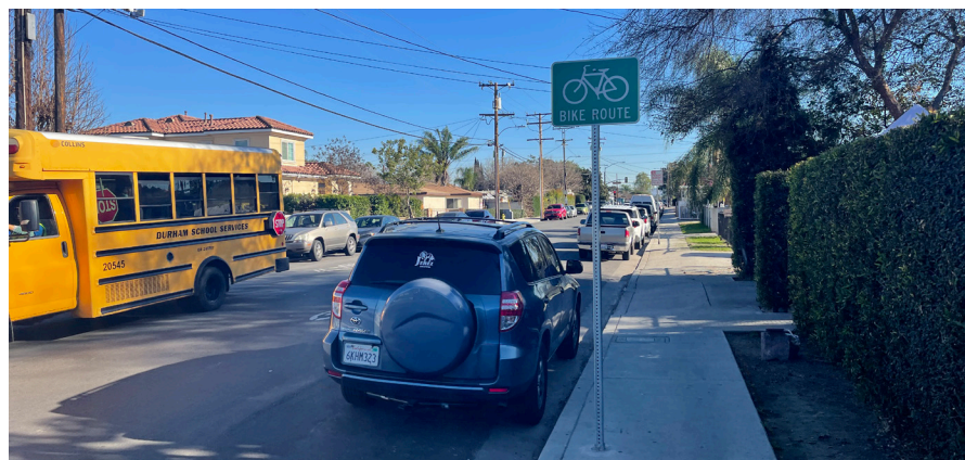
Existing roadway conditions along Magnolia Street
