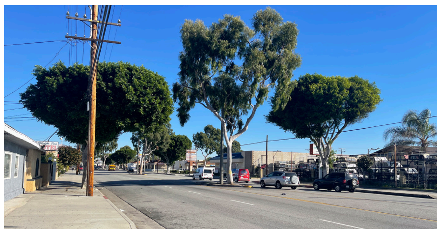
Existing roadway conditions along Garvey Boulevard
