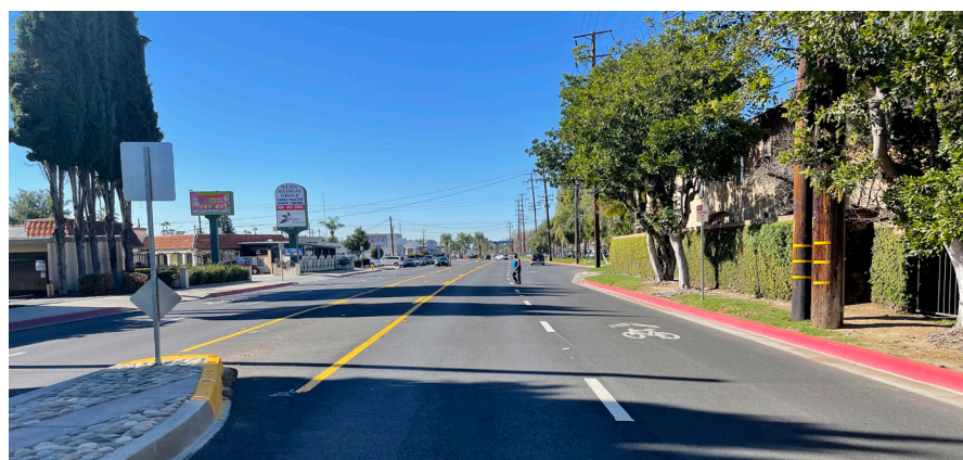
Existing roadway conditions along Ramona Boulevard
