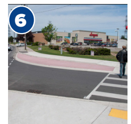
Corner Radius Reduction with Truck Apron
