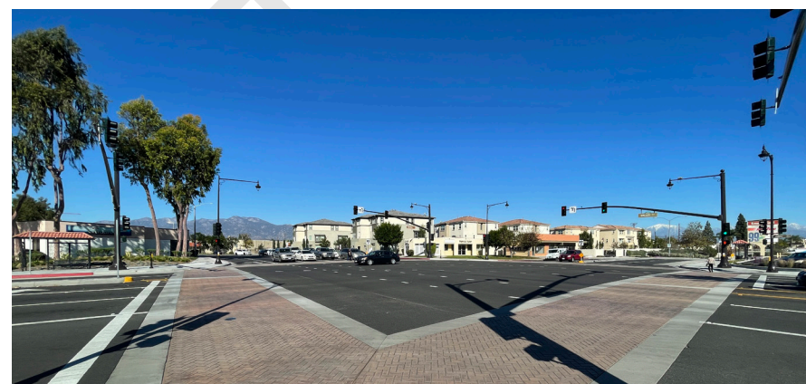
Crosswalks at Valley Boulevard and Ramona Boulevard
