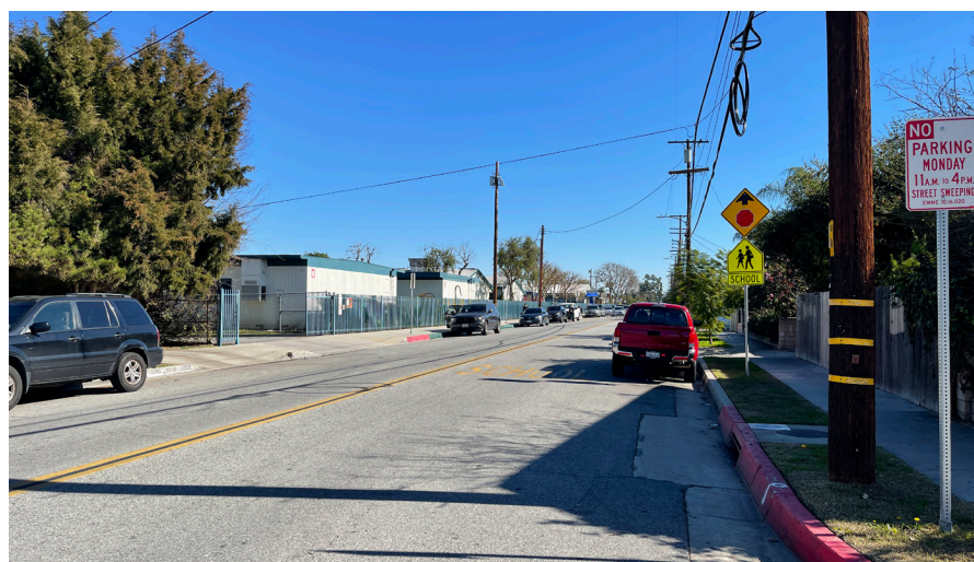
Existing roadway conditions on Bryant Road
