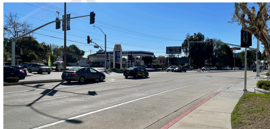
Installation of new traffic signal at McGirk Avenue
