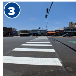
High Visibility Crosswalks
