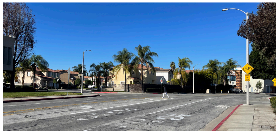
Existing roadway conditions along Tyler Avenue
