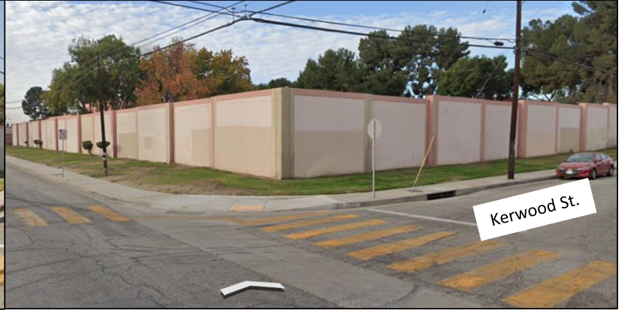
Looking south from corner of Kerwood and Gilman
