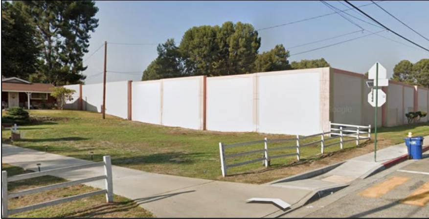
Looking north from Gilman at southern boundary of property
