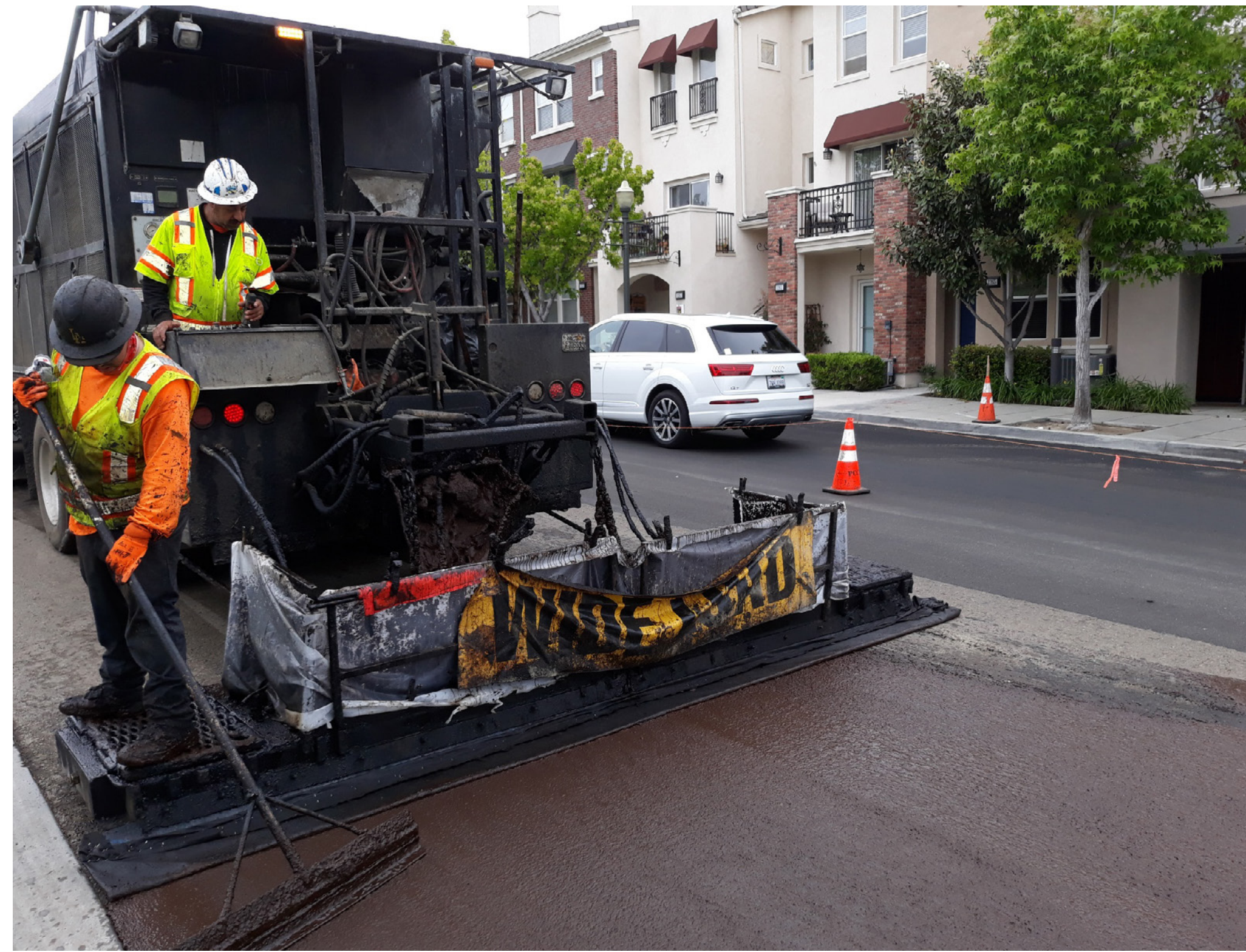
Slurry Seal
