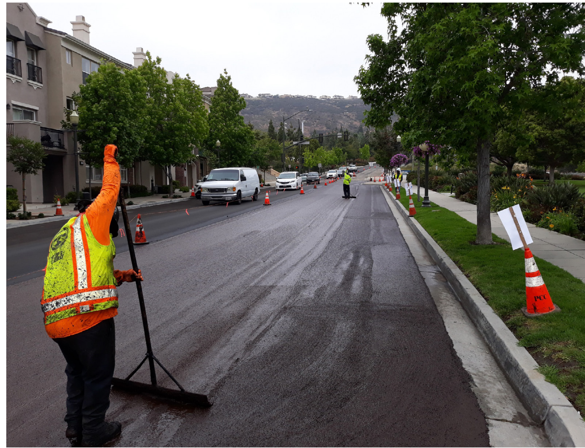
Slurry Seal
