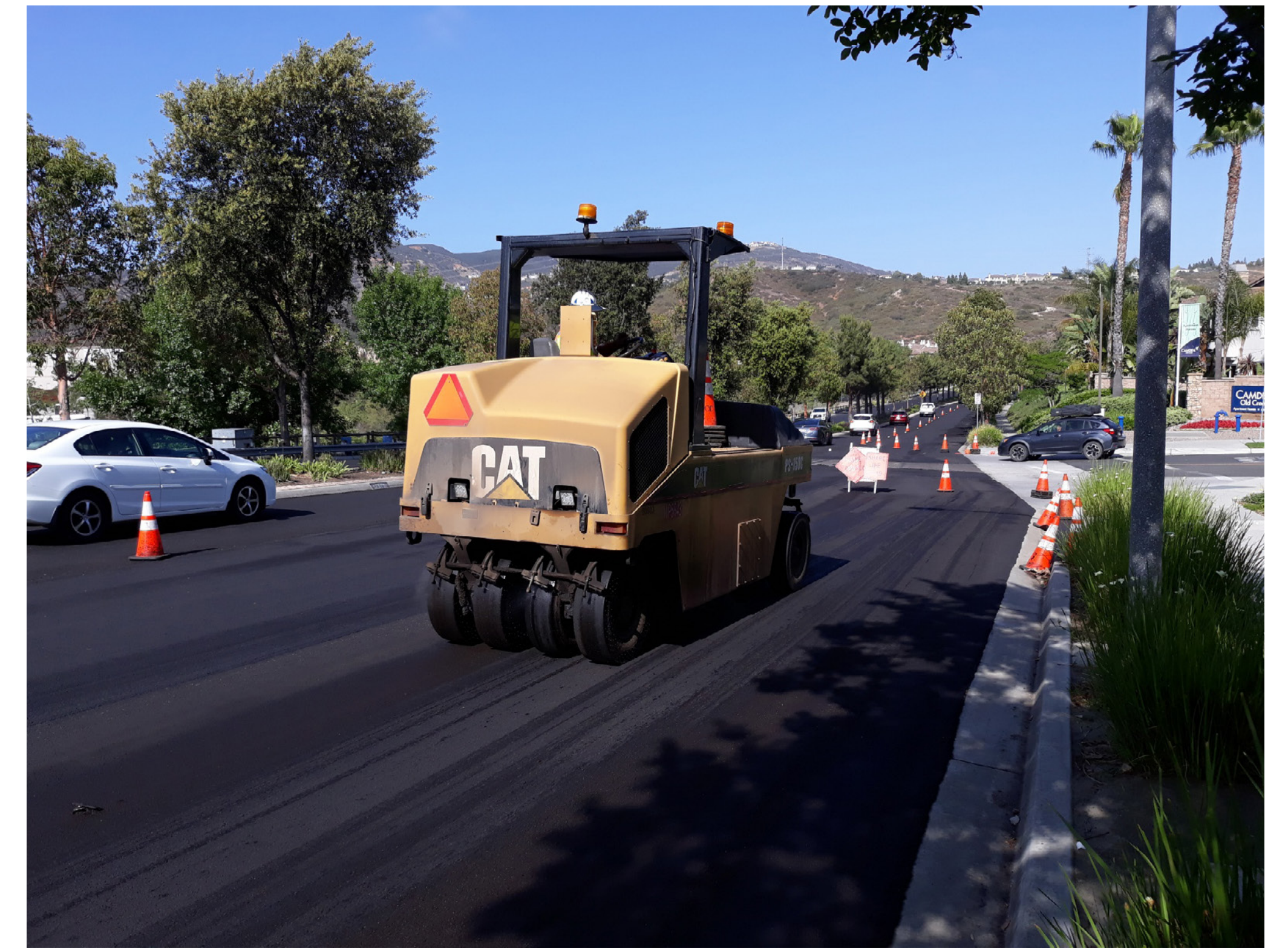
Slurry Seal
