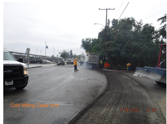
Grinding & Paving Operations Along Cedar Ave
