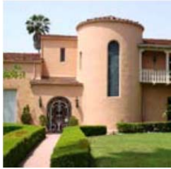
Complex Roof Forms
