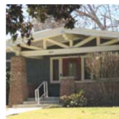
Exposed Beams and Rafters
